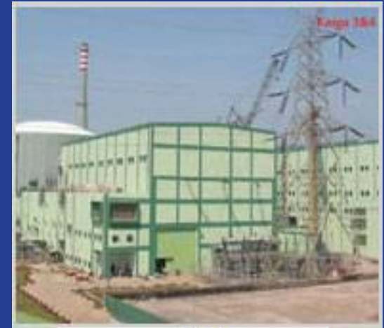
KAIGA ATOMIC POWER PROJECT
